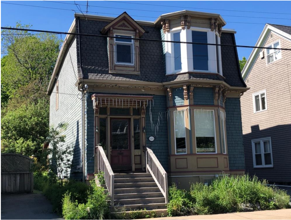
Figure 12: South and west façades
