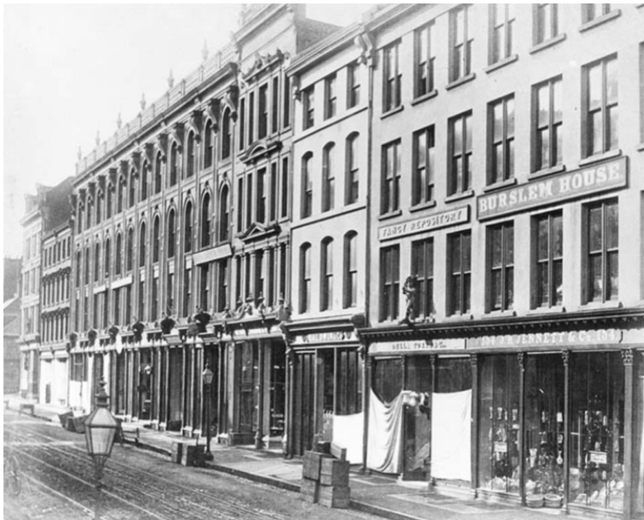
Figure 10: Baldwin & Co. at 148-150 Granville Street, undated (Source: Nova Scotia Archives)
