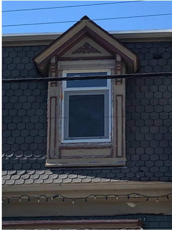
Figure 18: Gable dormer with projecting eaves on the south façade
