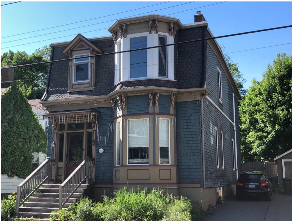
Figure 13: South and east façades
