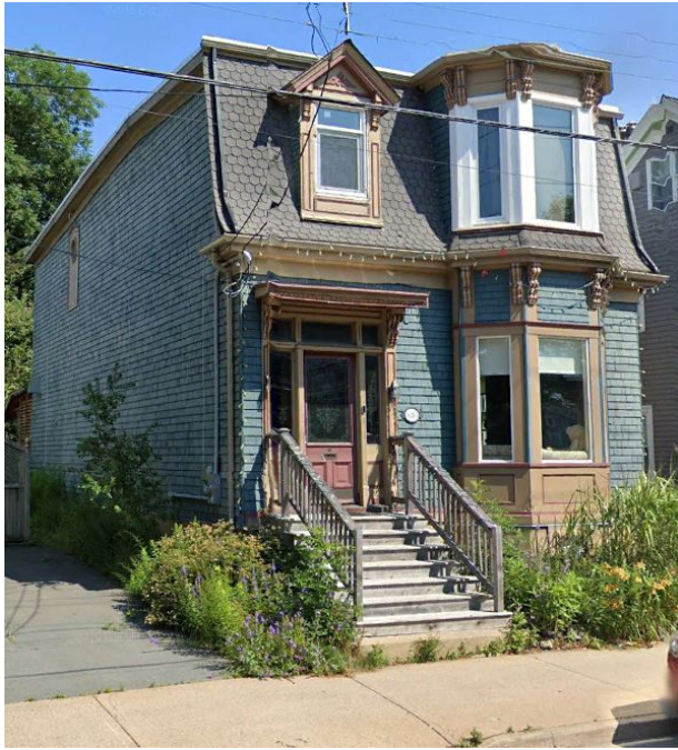
Figure 1: 6215 Coburg Road (Google Street View)
