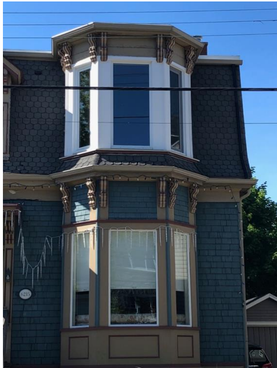
Figure 19: Two-storey bay window on the south façade
