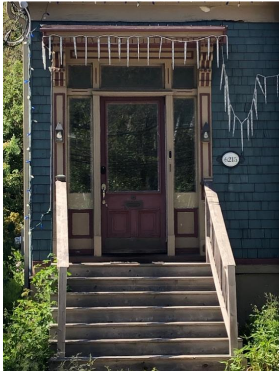
Figure 21: Single-leaf entrance with sidelights, multiple-light transom and entablature
