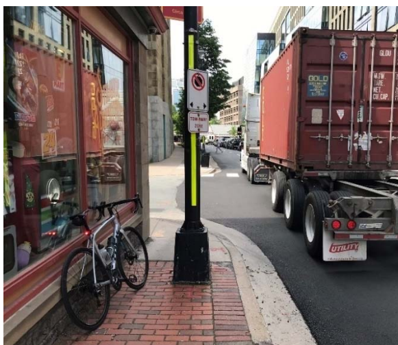
Photo 2: Looking north on Lower Water Street toward Prince Street. The street light pole at the intersection reduces the pedestrian clear width to 0.7m.
