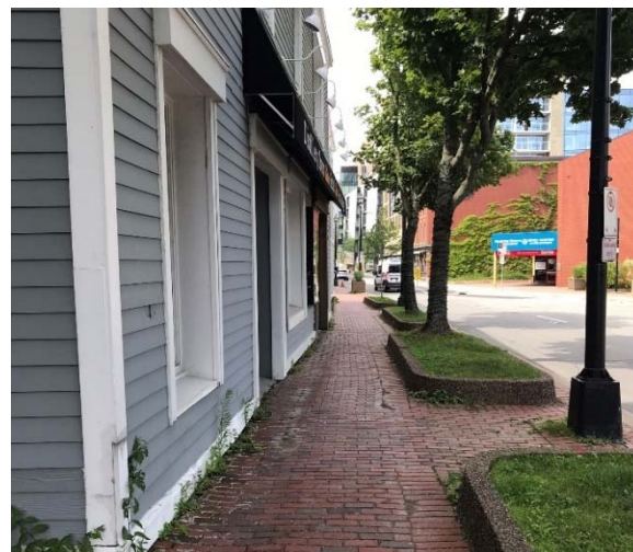
Photo 1: Looking north on Lower Water Street from Civic 1668. Raised planters reduce the pedestrian clear width to 1.5 – 1.9m.
