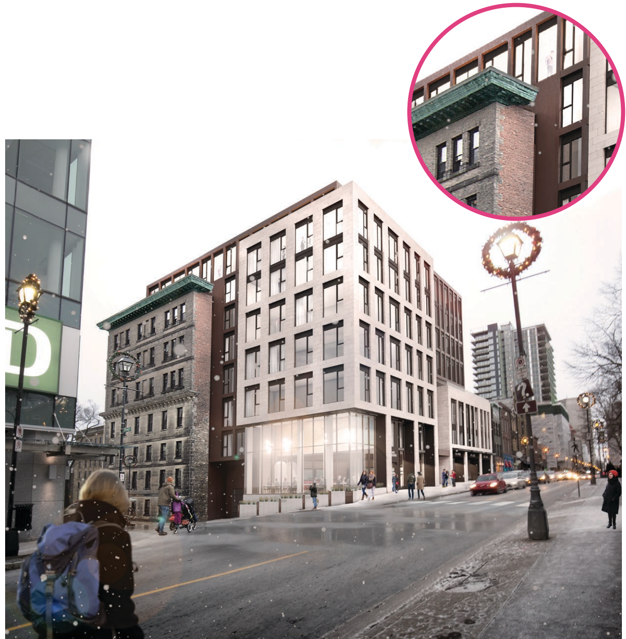
Figure 2.5.b Streetline Setback: Reveals at streetwall and retention of building returns allow for articulation of historic details.
