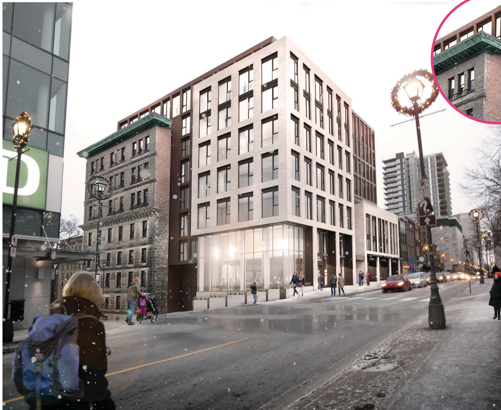
Figure 2.5.b Streetline Setback: Reveals at streetwall and retention of building returns allow for articulation of historic details.
