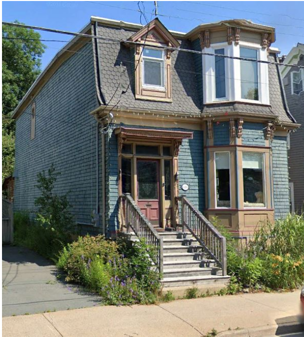
Figure 1: 6215 Coburg Road (Google Street View)
