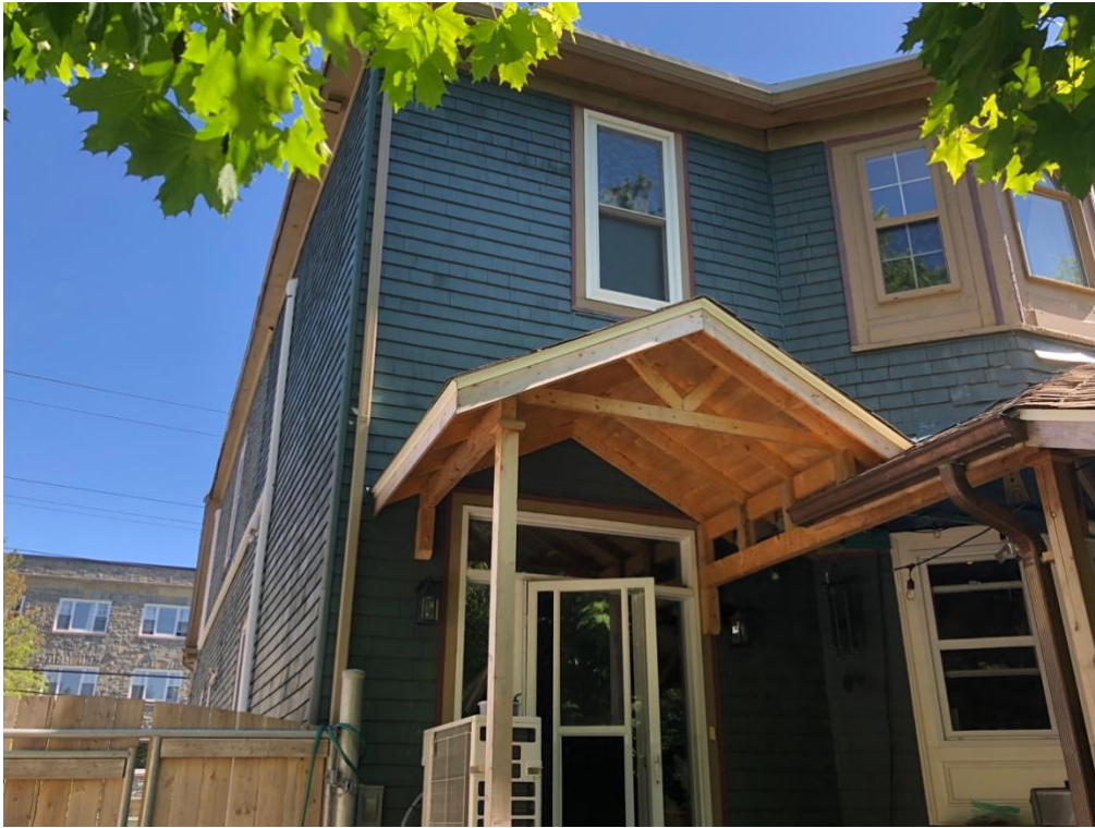
Figure 22: North façade entrance
