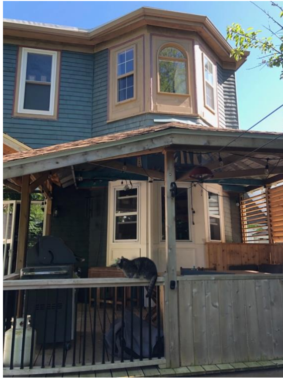
Figure 20: Two-storey bay window on the north façade
