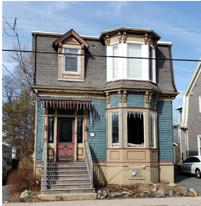
Figure 4: 6215 Coburg Road (Google Street View)
