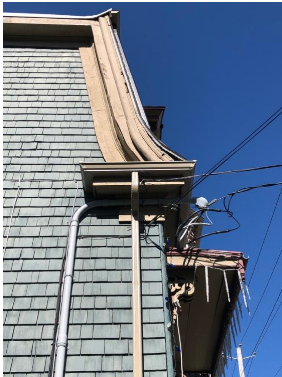
Figure 17: Mansard roof with returned eaves
