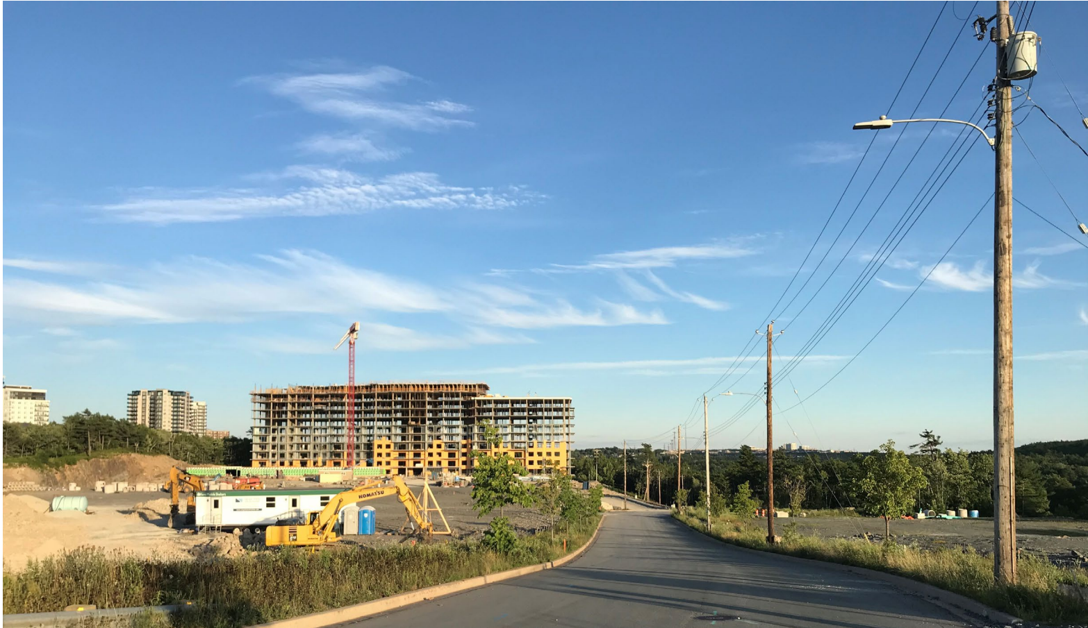
Looking southeast on Hogan Court
