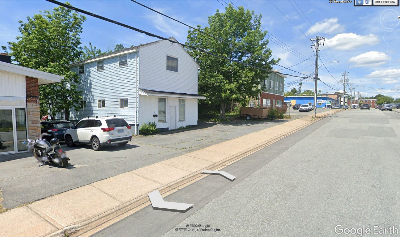
Subject site seen from Rosedale Drive looking towards Mitchell Street
