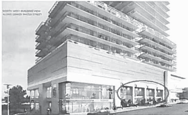
Figure 2 Lower Water St side of building. Design Manual requires storefronts on the streetwall. Instead there is 37 m of planters
