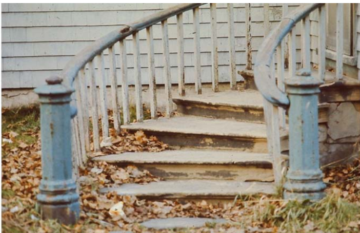
Cast-iron balustrades and newels and sandstone steps, 1974. 22
