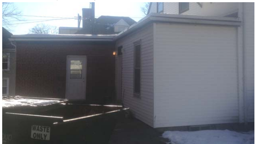
Rear of east addition
