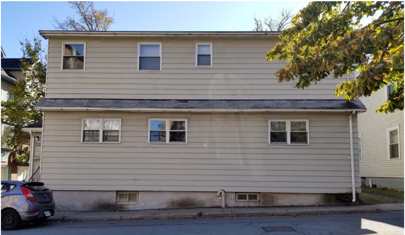
North, Harvey Street, elevation
