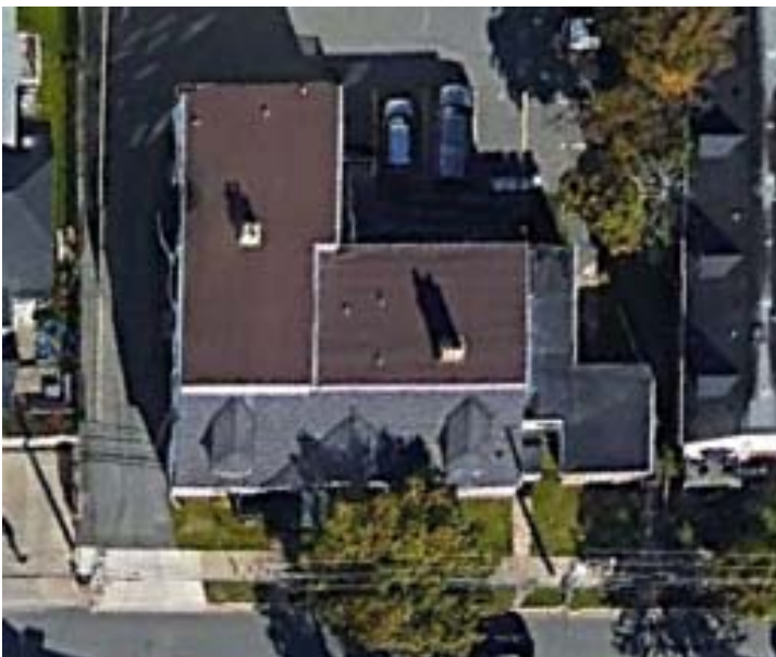
Existing building aerial view.
