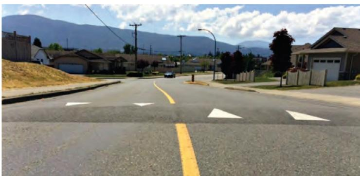
Speed Humps are traffic calming devices that use vertical deflection to slow motor-vehicle traffic in order to improve safety conditions.
