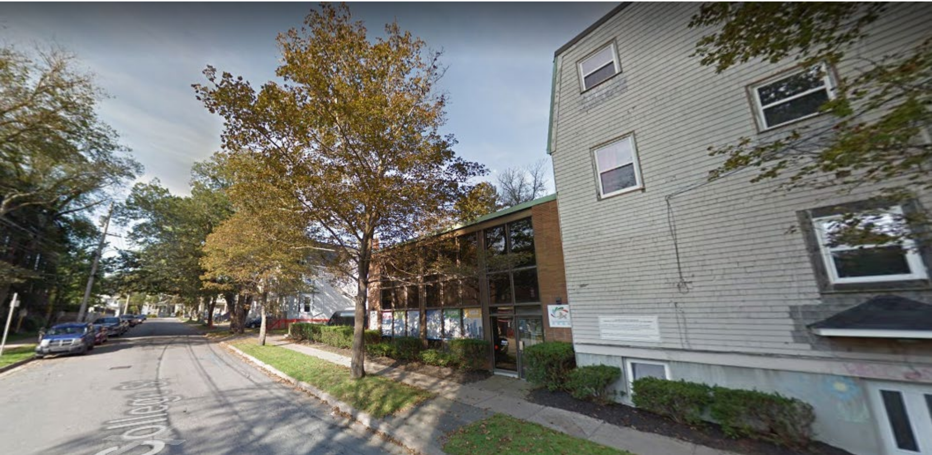
Subject site looking west from College Street.
