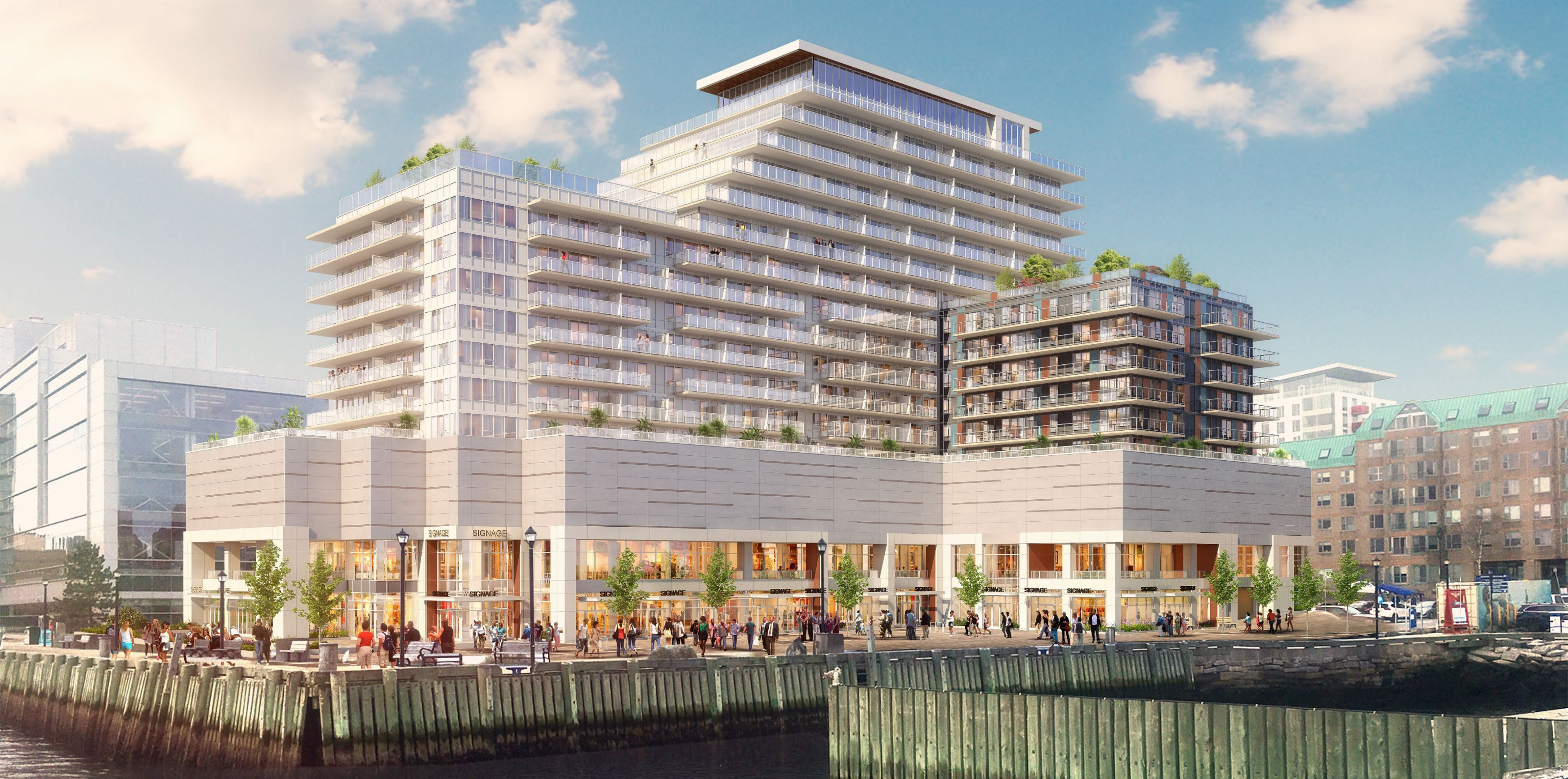
NORTH EAST VIEW ALONG THE PLAZA
