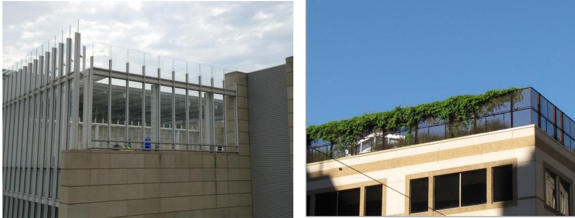
**Image 3 – Examples of Porous Parapets**
