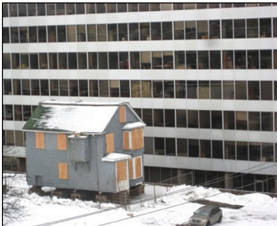
Figure 5: Morris House - 2009. Located on Nova Scotia power lands. Source: The Griffin, June 2013, 38, No.2 ISSN 0384 7335
