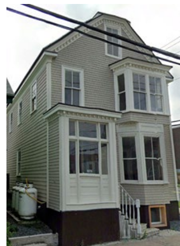
Figure 4: Current view of Morris House at its Creighton Street location
