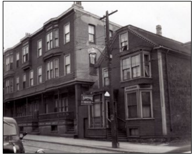
Figure 4: The Morris House at 1273 Hollis Street in April 1953 next to the Victoria Hotel. Source: The Griffin, June 2013, volume 38, No.2 ISSN 0384 7335
