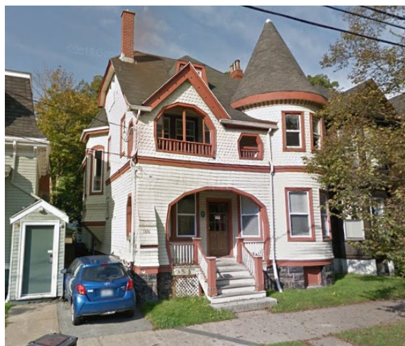
Figure 3. 1328 Robie Street (Another Harris-designed Dwelling)
