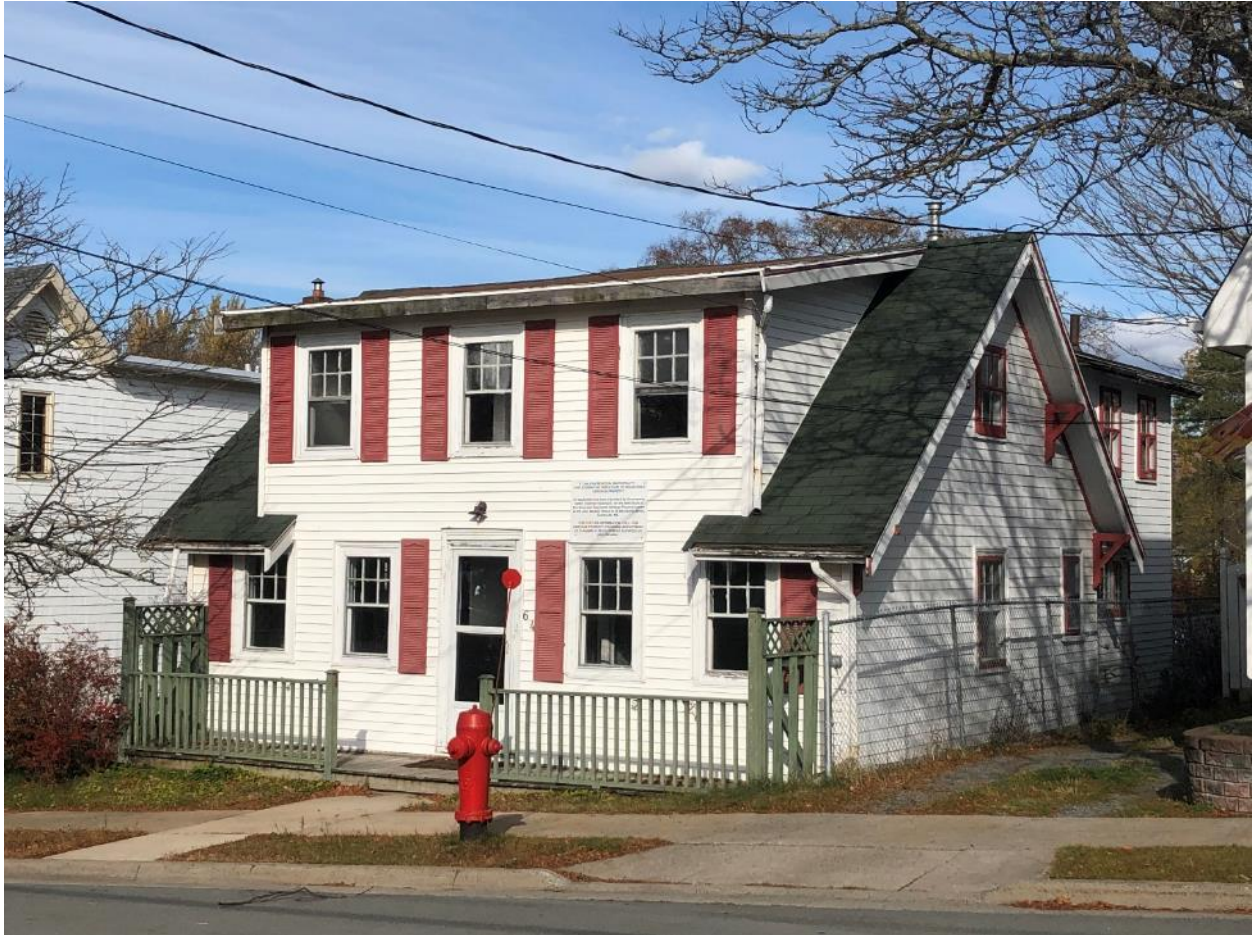
Figure 1: Front, south, elevation of the heritage building with large central dormer extending through the roof installed in 1962
