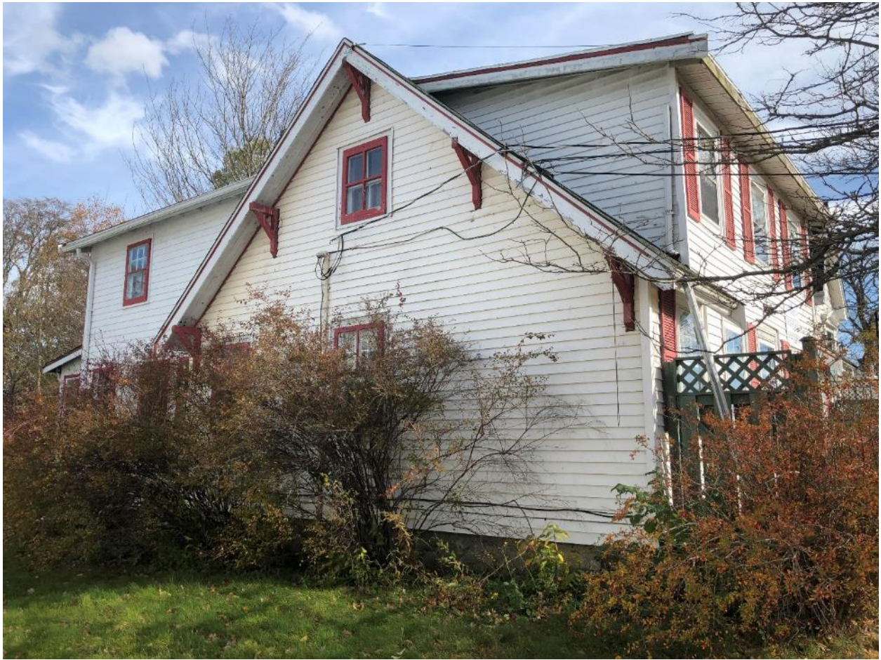
Figure 2: West side elevation showing steeply pitched gable roof with overhanging eaves supported by brackets installed in the 1960s
