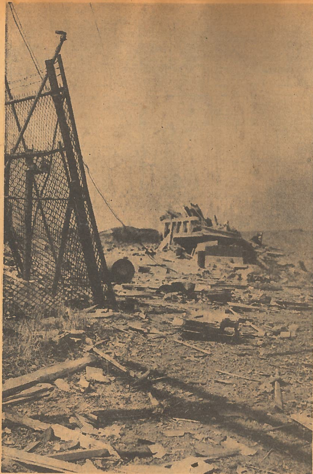
These Halifax Mail photos are the first taken inside the Bedford Magazine area after the explosions. Top picture shows the rubble left where buildings disappeared and below is a general view of the destruction.
