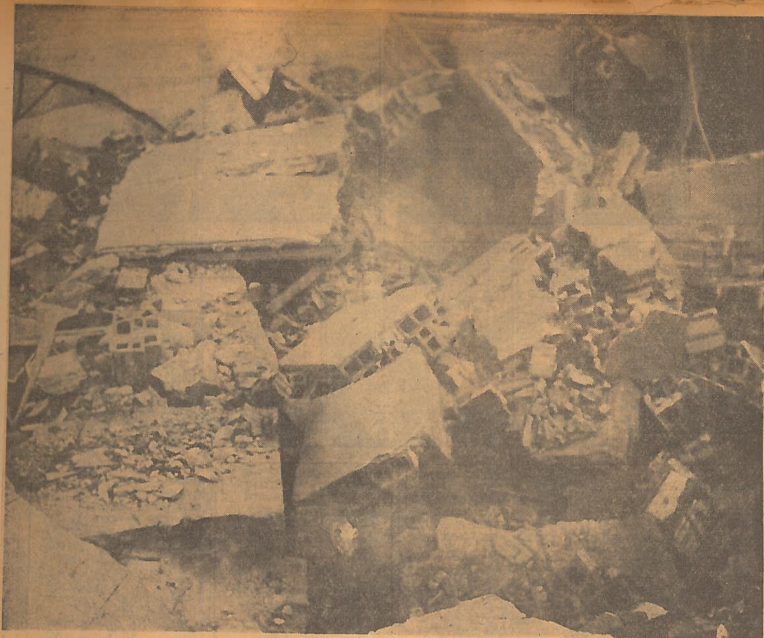
FIRST PICTURE —What the explosions did to strong buffers built to withstand blasts and protect other ammunition stores.
