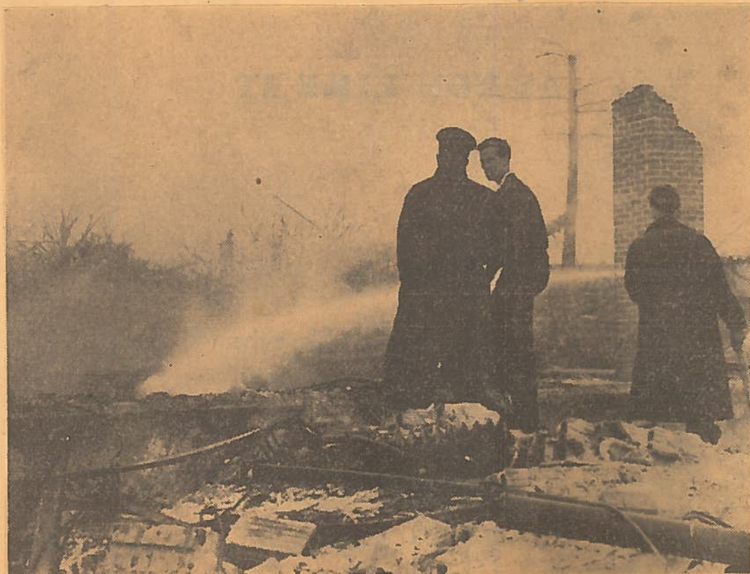
PLAY WATER ON FLAMES —Firefighters of the Navy this morning continued to pour water on the brush fires that started as a result of the Bedford Basin magazine explosions. Above, three of the firefighters are shown at the site of the staff house near what was the main gate of the magazine. (Photo by R. Allen Benjamin.)
