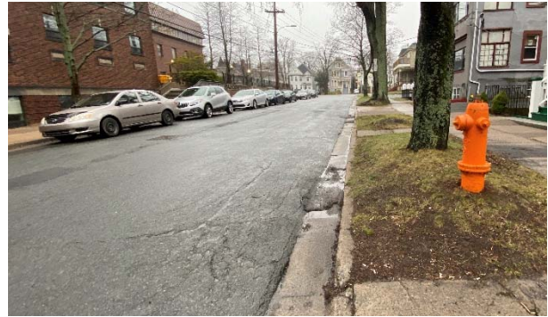
Photo 8 - Looking Right (West) on College Street towards Robie Street
