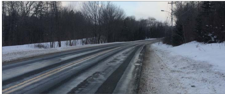
Photo 3: Looking west (to the right) on Windgate Drive from the proposed site access Intersection
