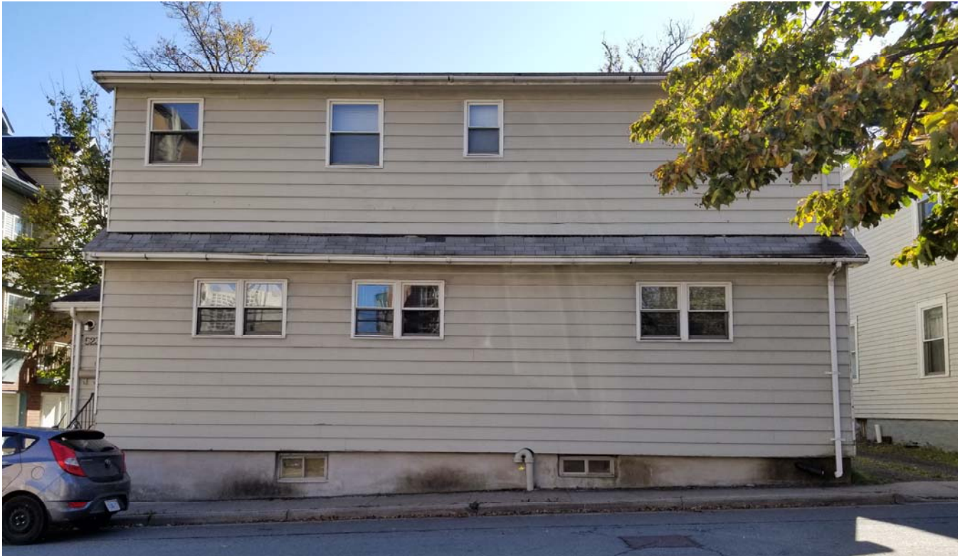
North, Harvey Street, elevation
