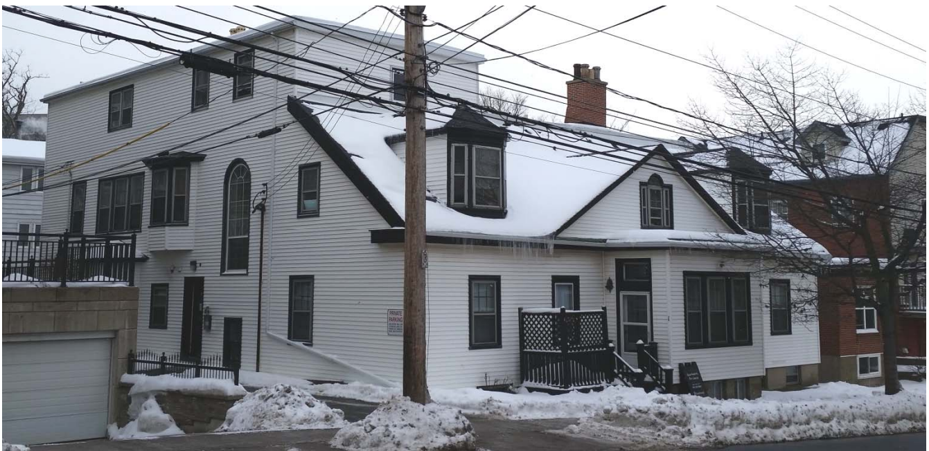
Street view from the southwest showing rear wing with third floor addition
