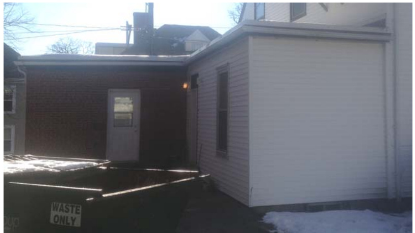
Rear of east addition
