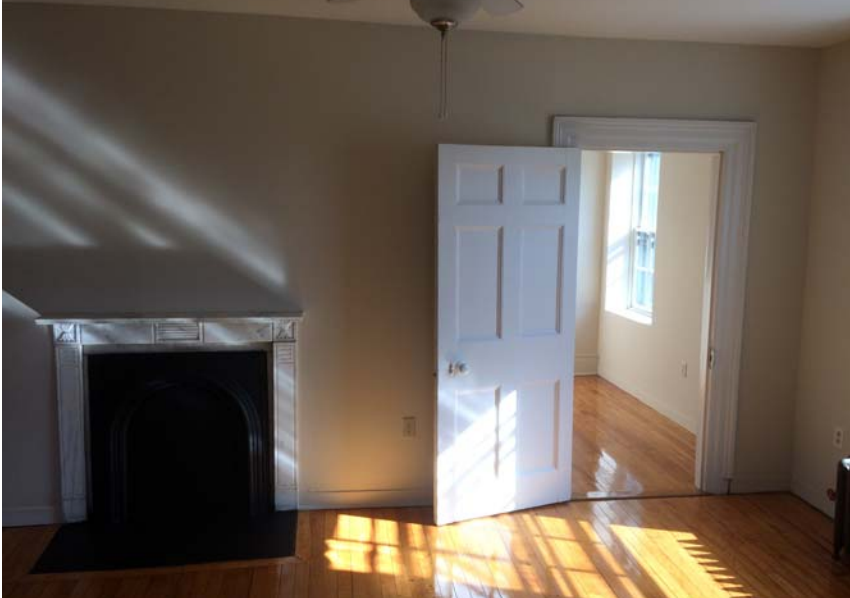
Upper floor south-east unit, south fireplace
