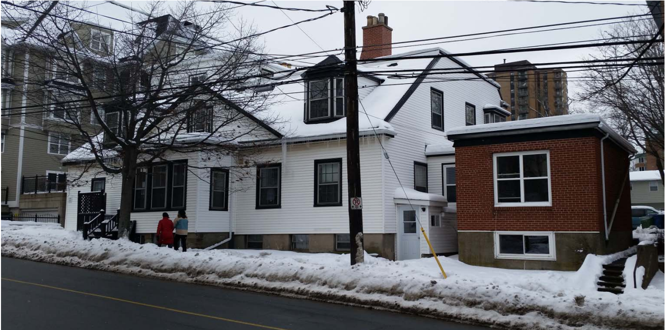
Street view from the southeast showing later one storey additions
