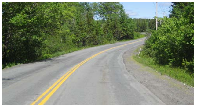
Photo 4: Westbound approach to proposed site access location. Note the trees obstructing sight lines on the right side of the photo.
