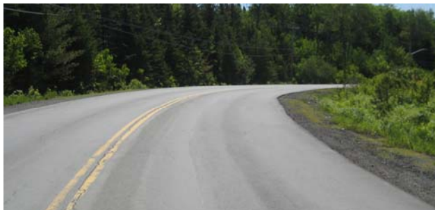
Photo 3: Eastbound approach to proposed site access location. Note the trees obstructing sight lines on the right side of the photo.
