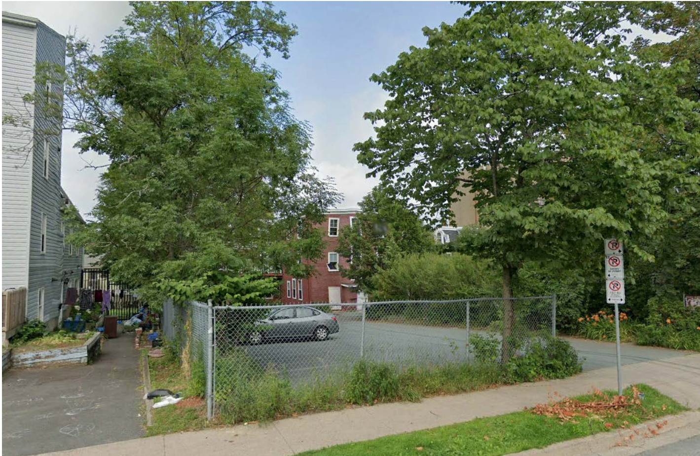
Subject Property from Creighton Street
