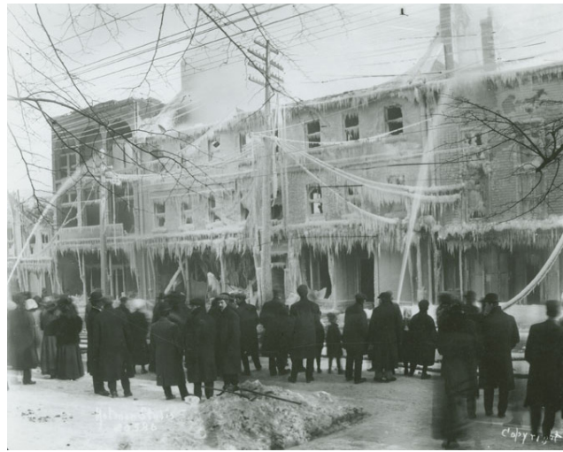
Fig. 4 1912 Barrington Street, looking east
