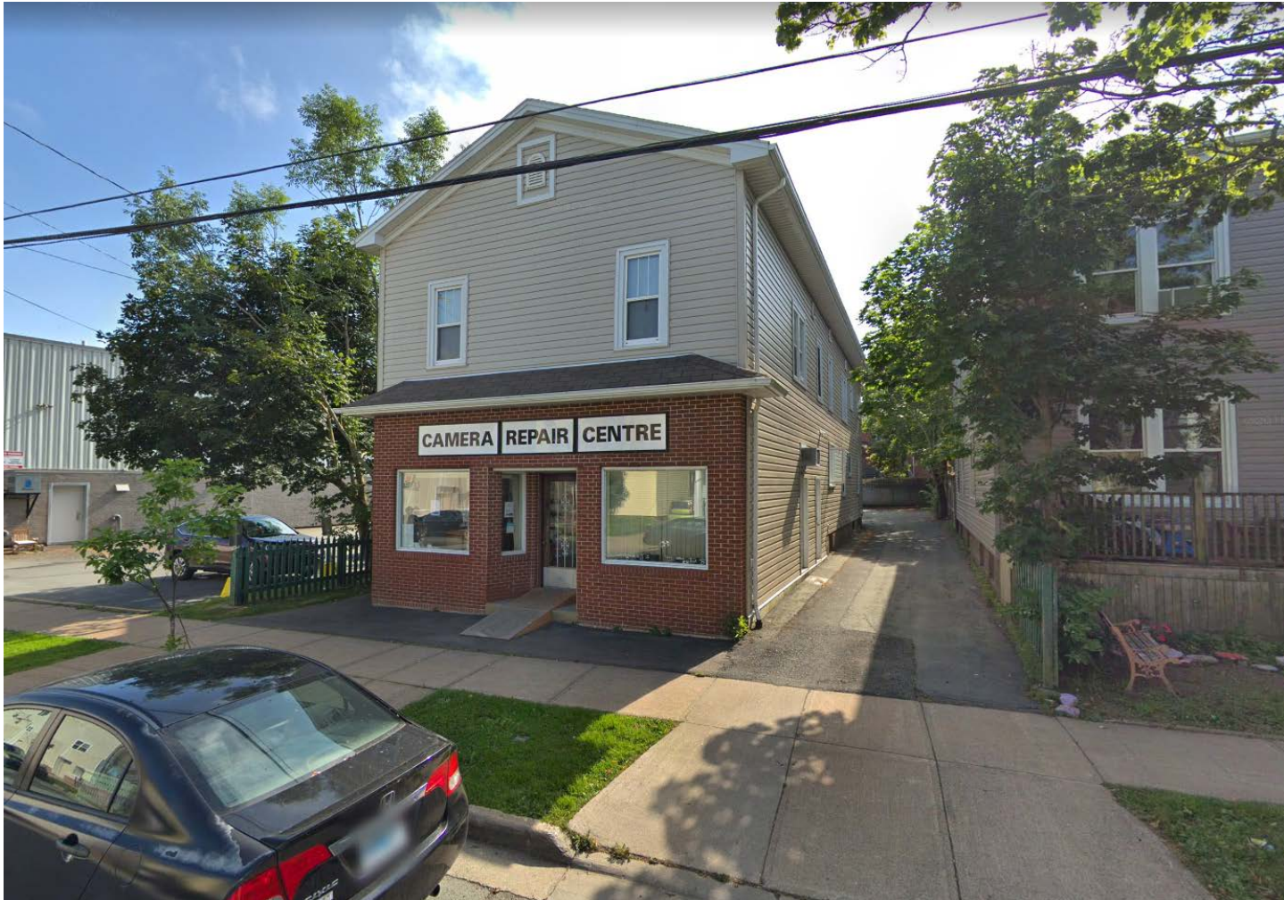
Subject site- side yard
