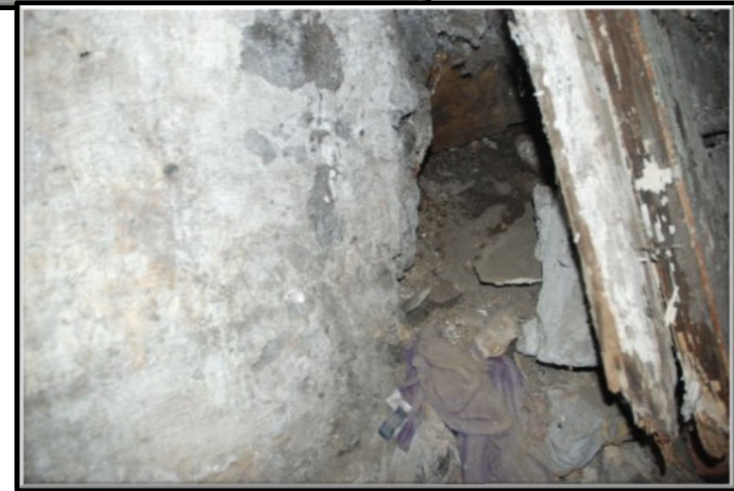
Detail of door used to retain earth at basement wall
