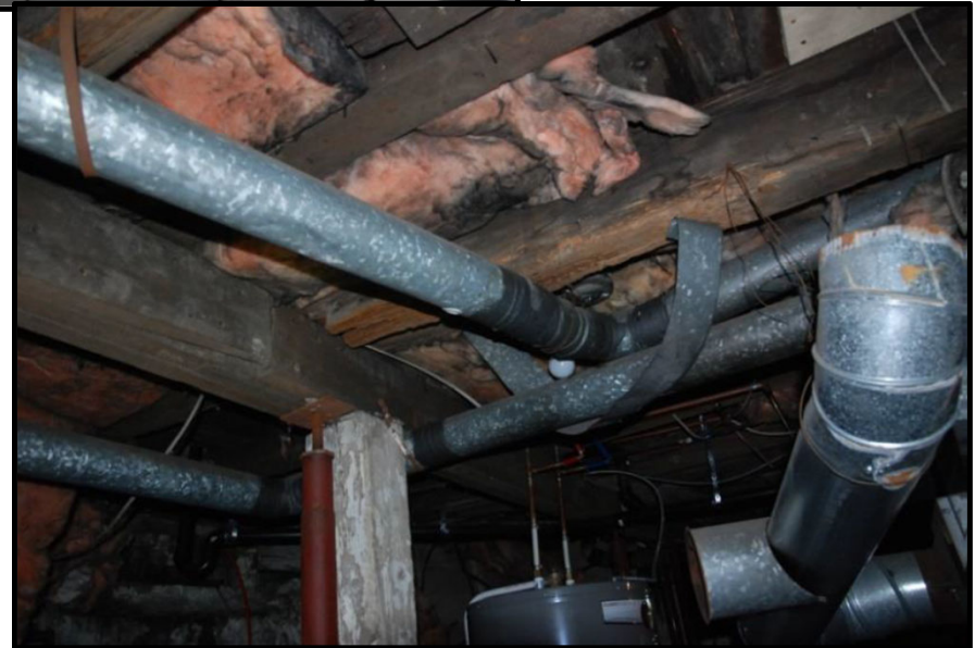
Decayed main floor framing with reconstructed main beam on post and jackpost
