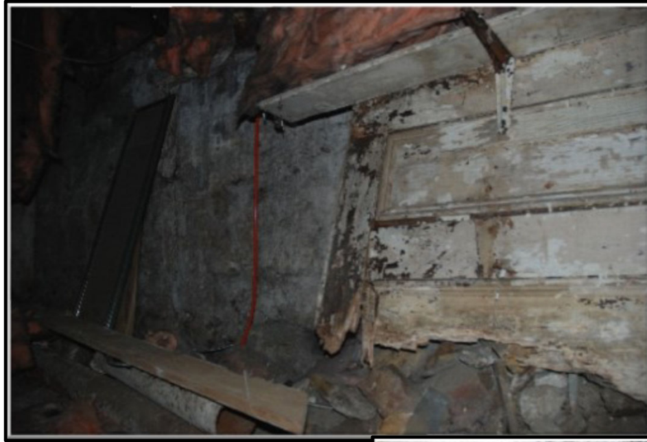
Door used to retain earth at basement wall
