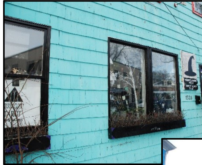
Detail of first floor replacement window
