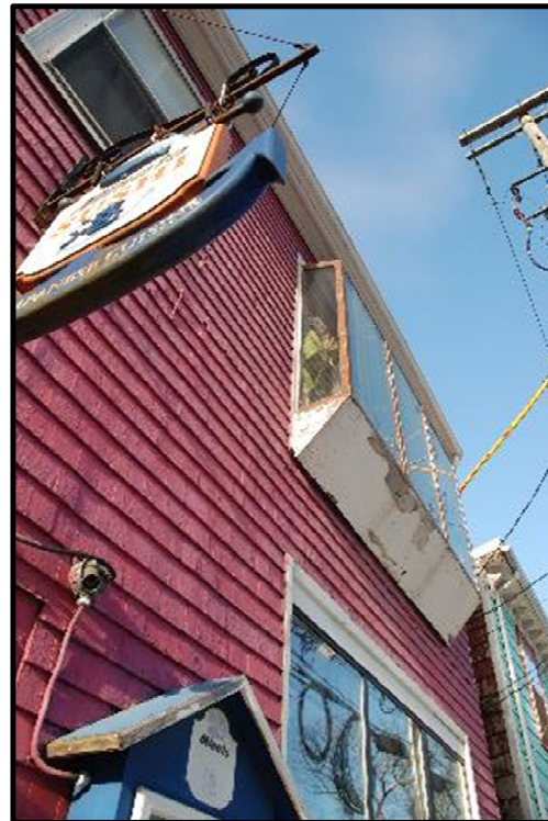
Detail of second floor bay window addition
