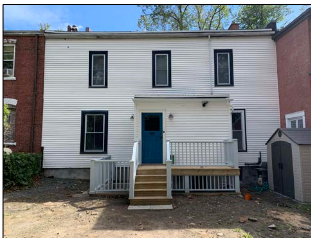
Figure 5: The rear of the building remains clad in white vinyl siding (Photo Sarah and Ian Bezanson)
