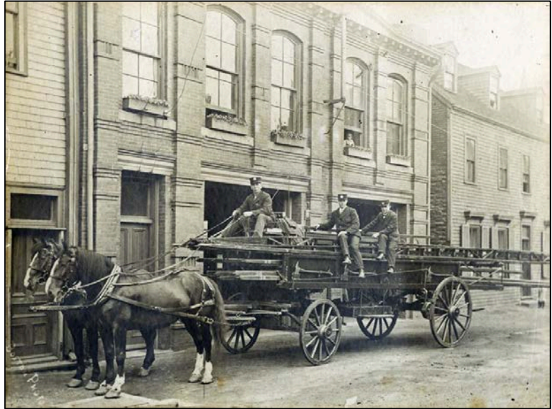
Figure 11: Photograph of 1579 Grafton Street, the No. 7 Fire Station, 1921. (Source: HRM).
