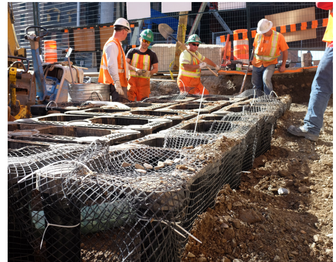
Example 3: Soil cells support healthy trees.
