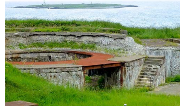
FIGURE 2: THE FORMER BATTERY AND GUN EMPLACEMENTS SURROUNDED BY THE NOW HARTLEN POINT FORCE GOLF COURSE.
