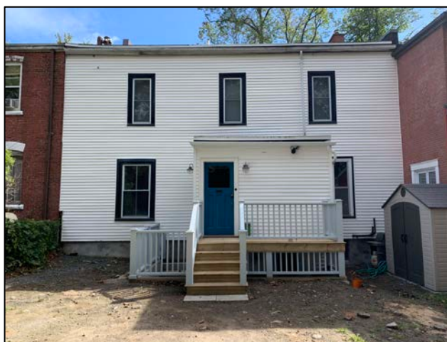
Figure 5: The rear of the building remains clad in white vinyl siding (Photo Sarah and Ian Bezanson)
