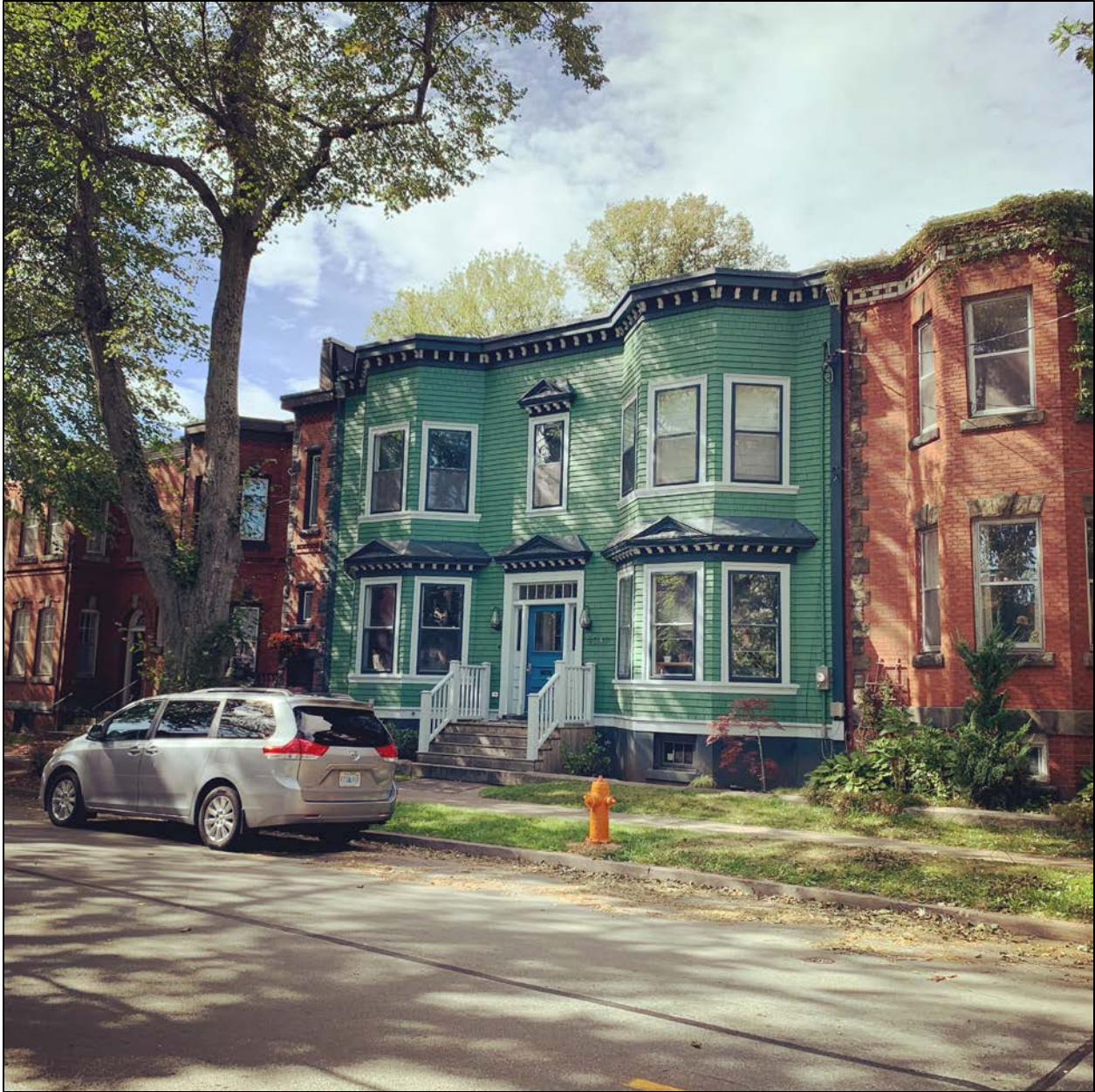
Figure 1: 6047 Jubilee Road was the first building constructed of the six rowhouses. It was originally a detached wooden one-and-a-half storey homestead with a gable roof before Edward Maxwell converted it into its current form to integrate it with the rowhouse development. (Photo: Sarah and Ian Bezanson)
