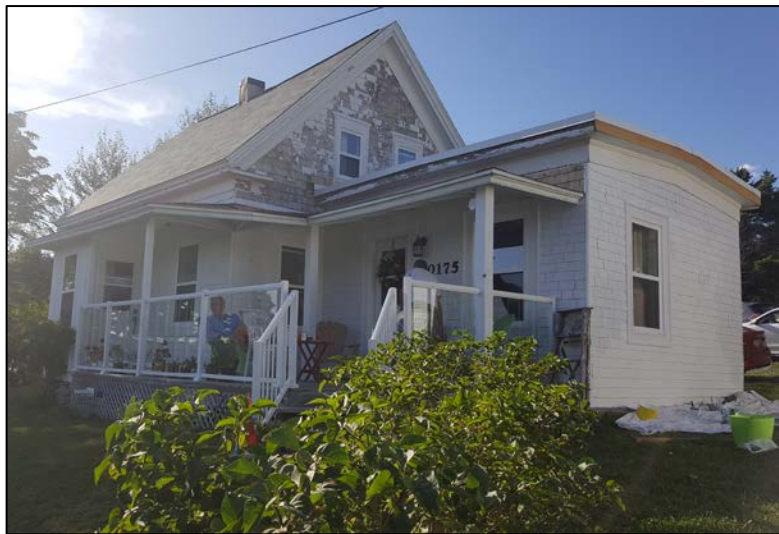
Figure 4: Photo of 10175 Highway 7 in 2019 (Image provided by Derek Thurber)
