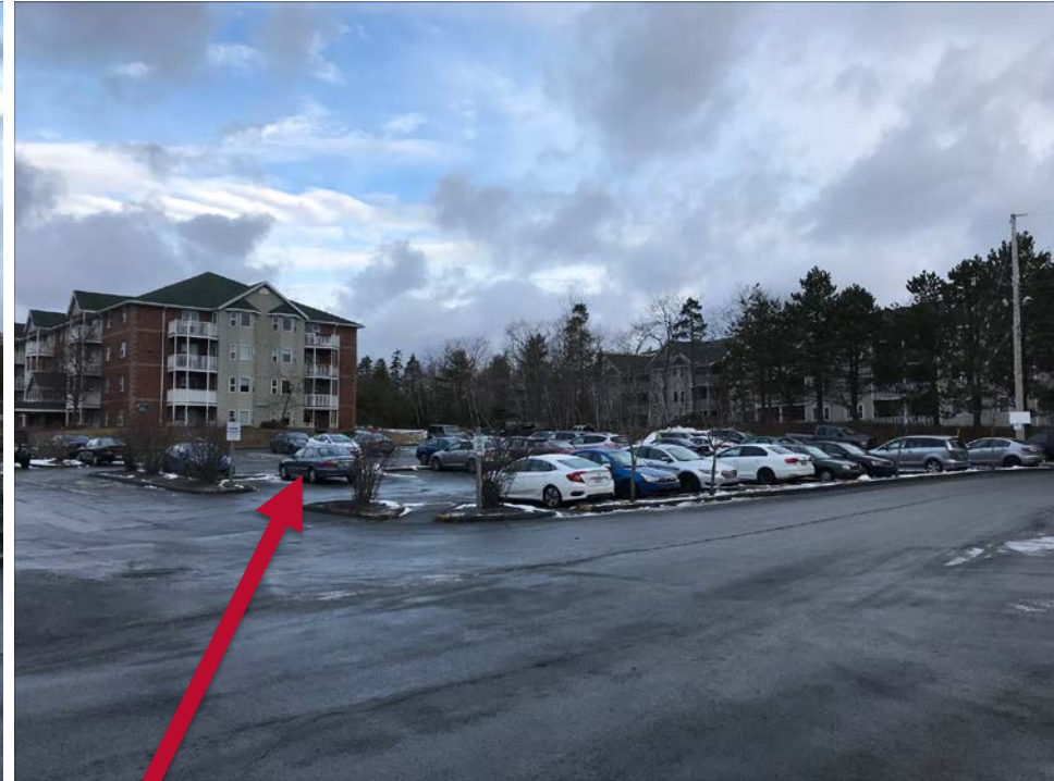
Area of 7-Storey Addition
