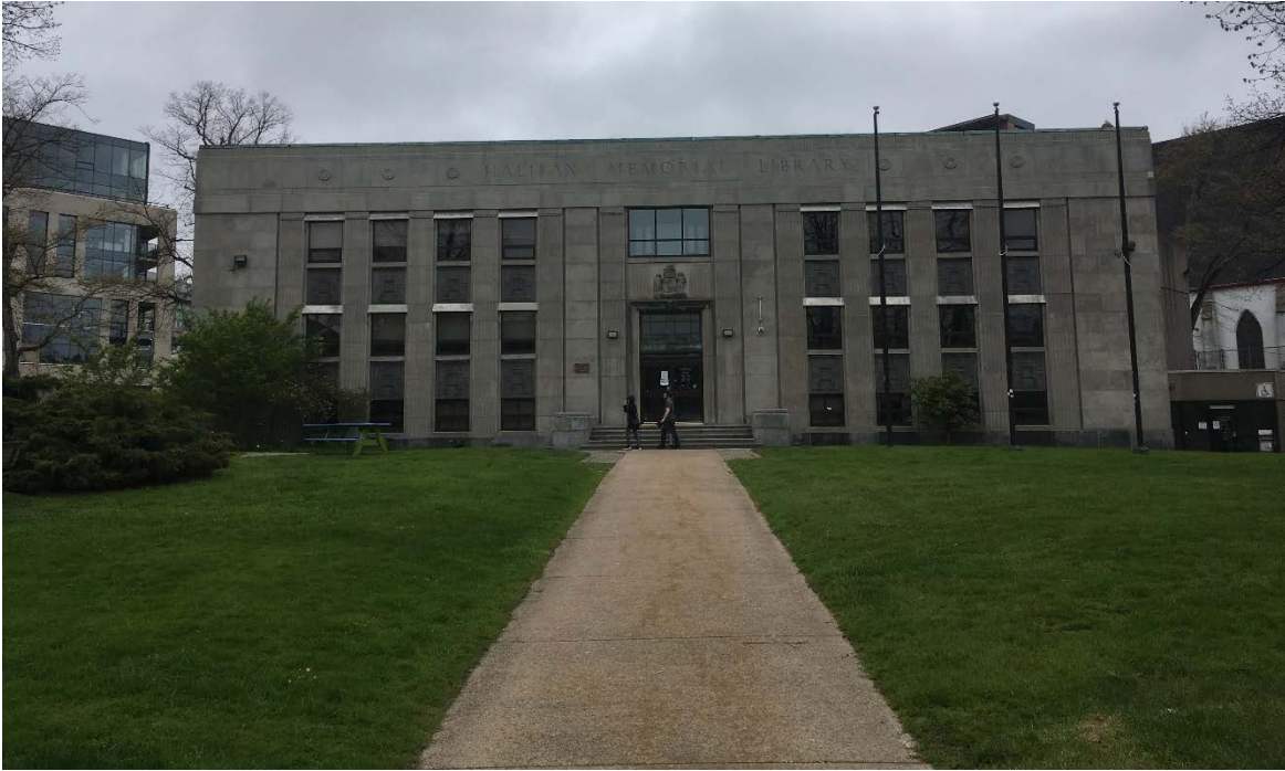
Figure 1 Former Memorial Library looking west from Grafton Street
