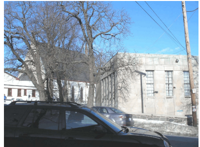
St. David’s Church and Memorial Library (rear) from Brunswick Street.
