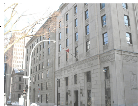
Dominion Building & Bank of Nova Scotia
