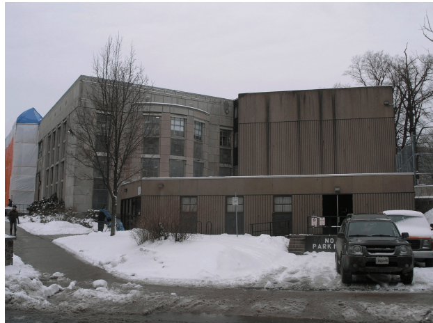
Addition: Front section viewed from Grafton Street.
