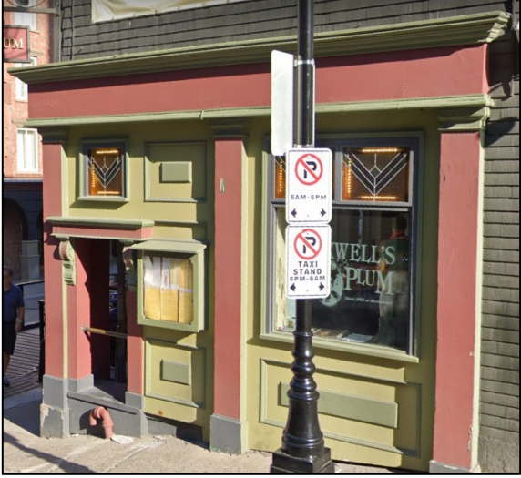
Figure 16: Side view of the storefront facing Sackville Street with the second doorway access near the corner of the lot, 2018. (Source: Google).
