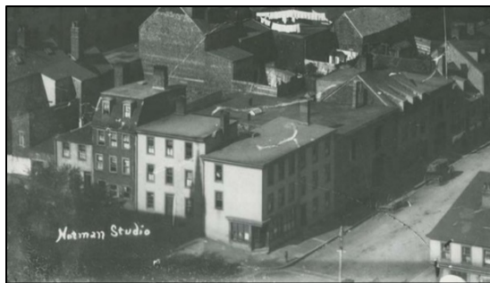
Figure 5: Lot 9 in 1888, depicting 1560 Grafton Street very close to its existing appearance. (Source: NSARM).
