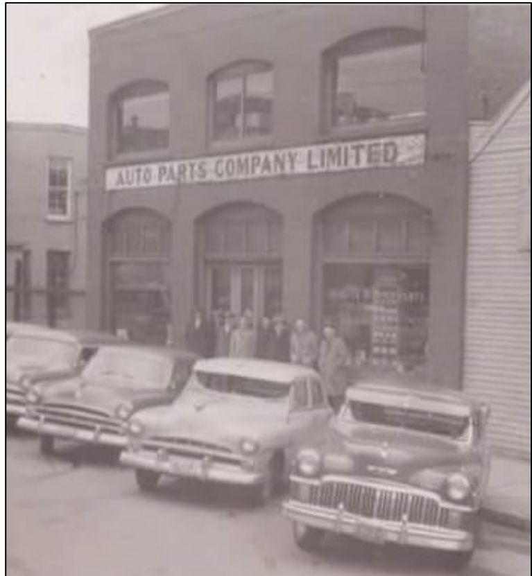
Figure 12: Photograph of 1567 Grafton Street in 1954 operating as Auto Parts Company Ltd. (Source: Unknown)
