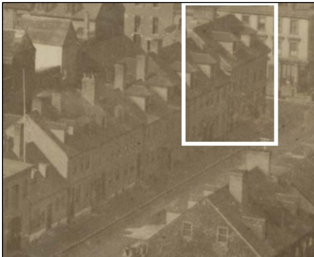
Figure 10: Photograph of the property. Note the Scottish dormers and central chimneys, 1888. (Source: NSARM).
