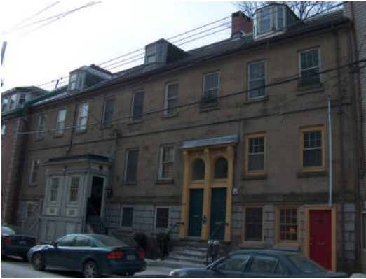
Three-bay building widths of Pryor Terrace on Hollis Street with side-hall plans
