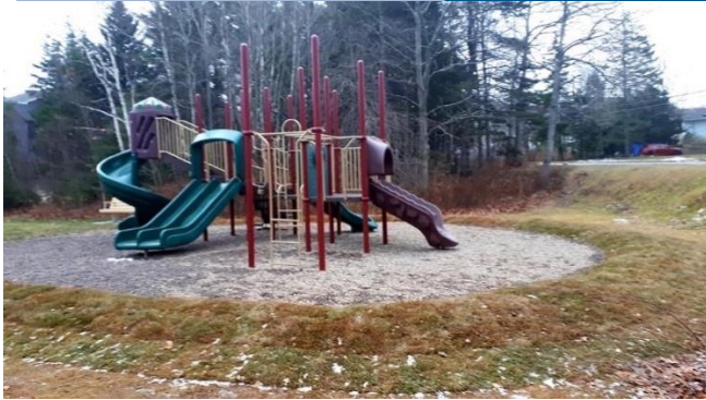
New berm around the playset at Belvedere Park replacing the old rotten wood framing.
