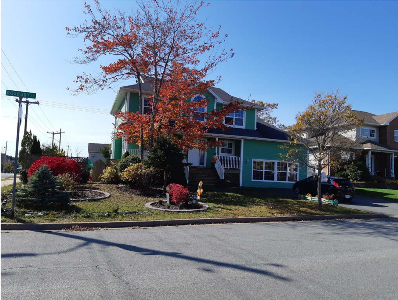
Subject site seen from the Roxbury Crescent
