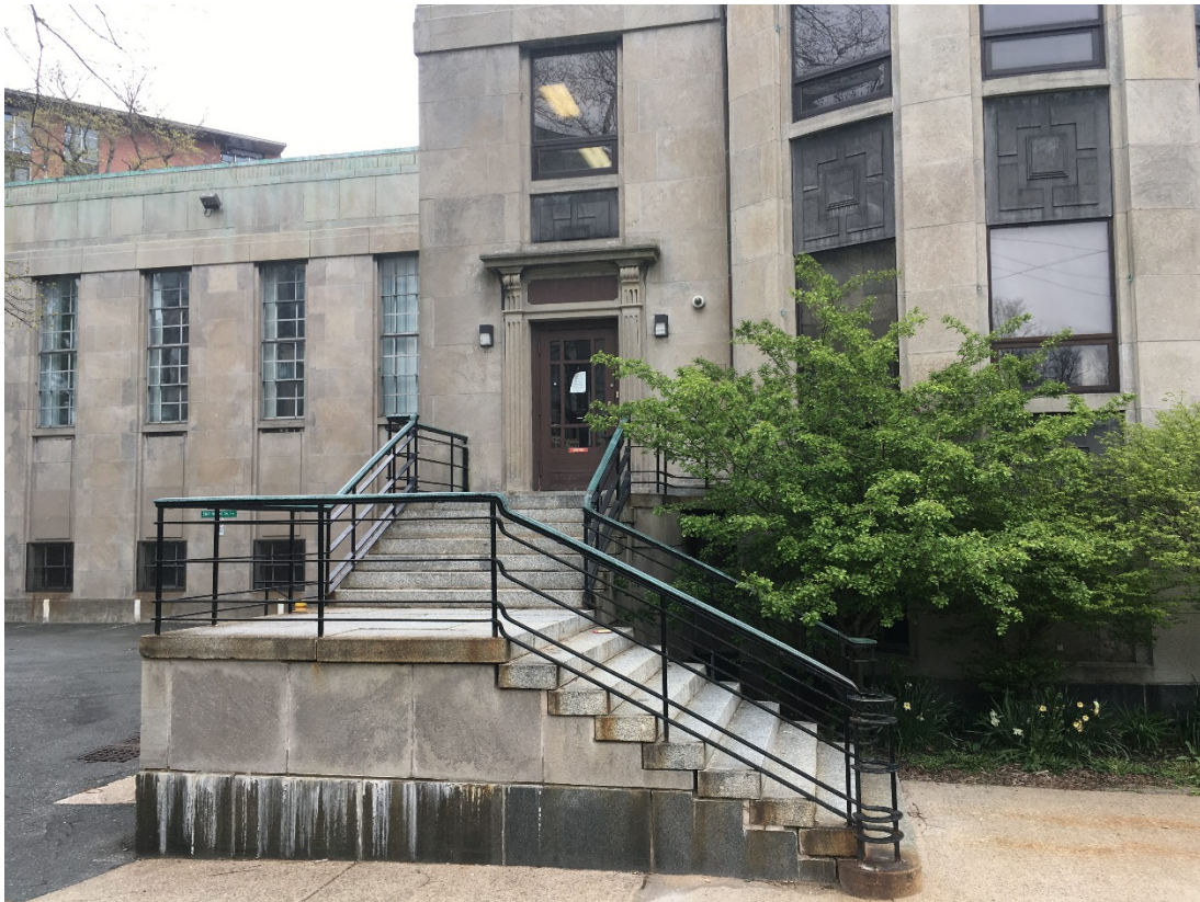
Figure 4 South entrance steps looking north
