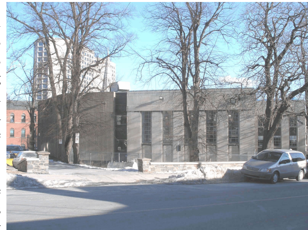
Addition: Rear section viewed from Brunswick Street.
