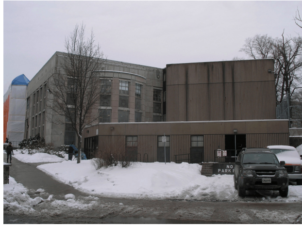
Addition: Front section viewed from Grafton Street.
