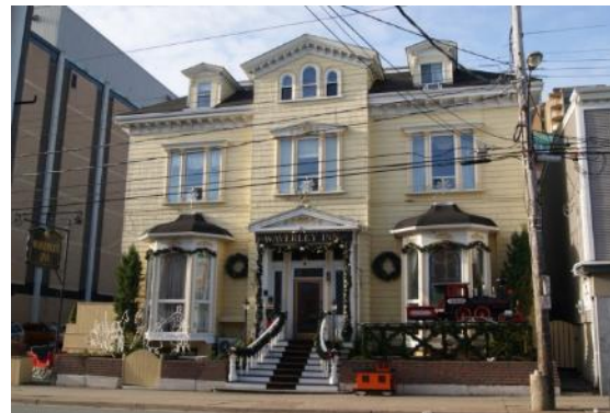
Waverley Hotel on Barrington Street with side yard and alley between neighbouring buildings
