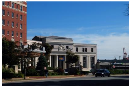
Canadian National Railway (Via Rail) Station with symmetry, classical detailing, and a 25-metre setback from the street
