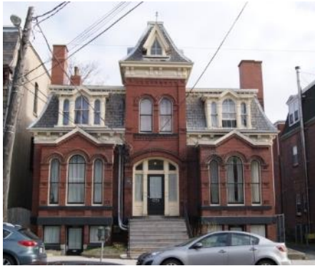
Renner-Carney House on Barrington Street with decorative brick corbelling
