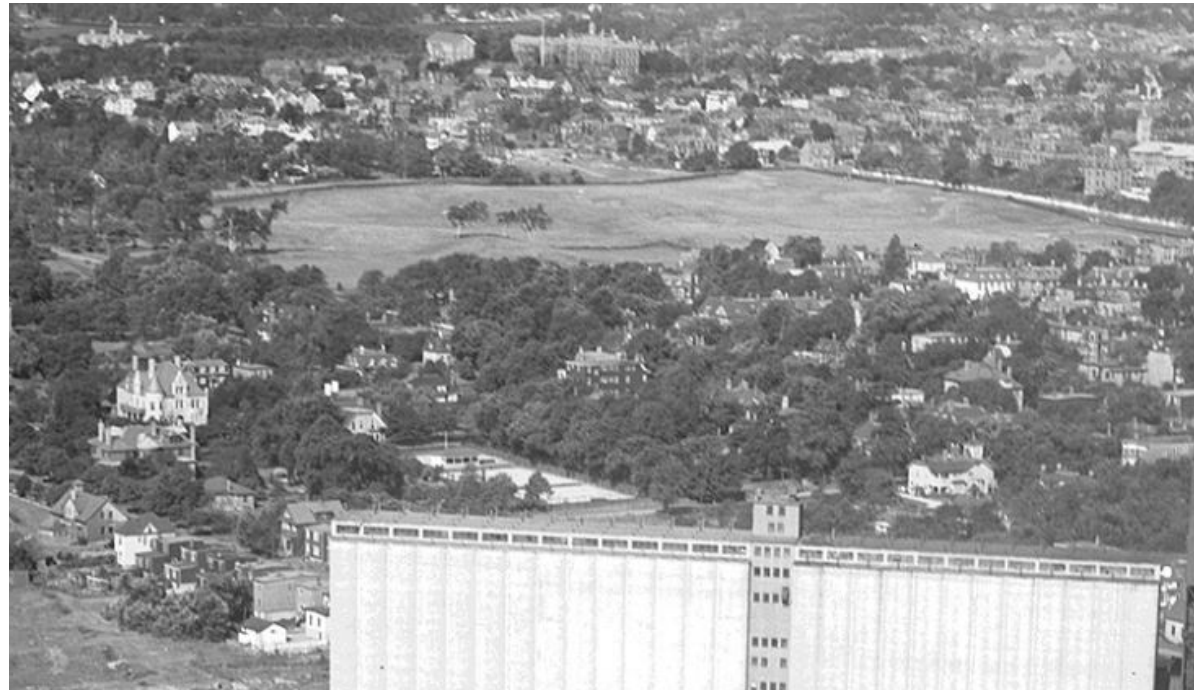
FIGURE 2: GORSEBROOK GOLF COURSE (NOW GORSEBROOK PARK) AERIAL PHOTO AS SEEN FROM HALIFAX HARBOUR, 1931.
