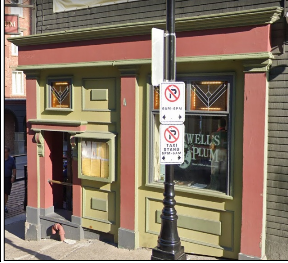
Figure 16: Side view of the storefront facing Sackville Street with the second doorway access near the corner of the lot, 2018. (Source: Google).
