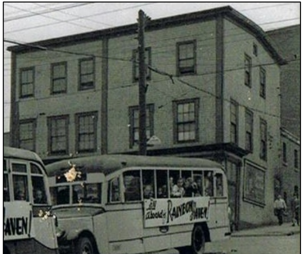
Figure 9: Photograph of the property in the late 1930s. (Source: HRM).
