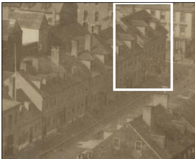
Figure 10: Photograph of the property. Note the Scottish dormers and central chimneys, 1888. (Source: NSARM).
