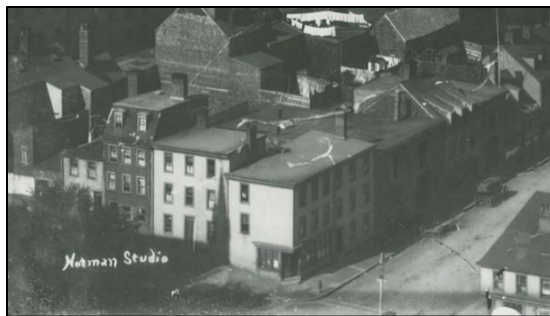
Figure 5: Lot 9 in 1888, depicting 1560 Grafton Street very close to its existing appearance. (Source: NSARM).
