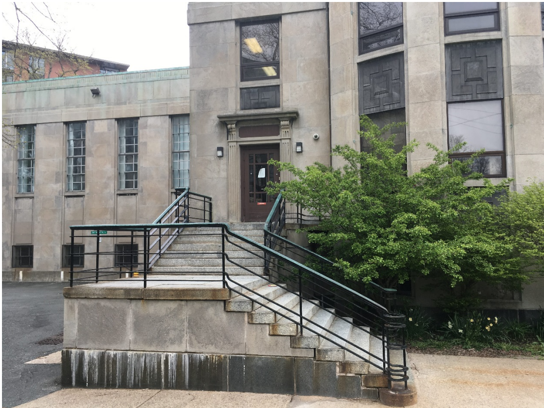
Figure 4 South entrance steps looking north
