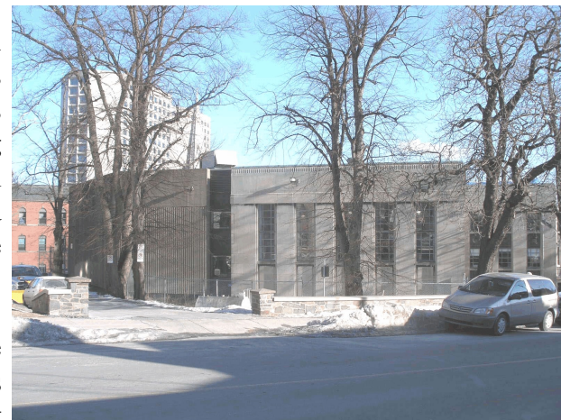
Addition: Rear section viewed from Brunswick Street.
