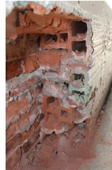
Speed tile on the interior of the brick, destructive testing
