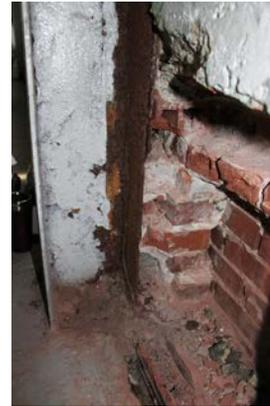
**Rusting on embedded structural columns due to moisture penetration through the masonry**
