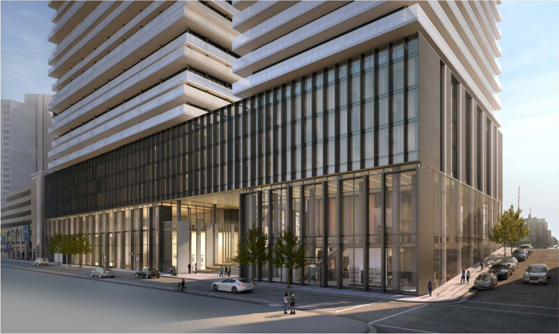
LOUIS STREET / SACKVILLE STREET VIEW
