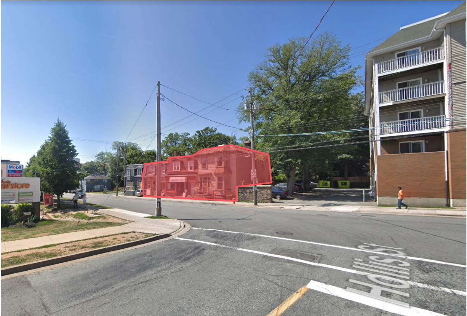
Subject site seen from Barrington Street and Hollis Street)
