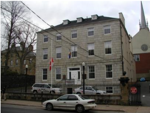
Black-Binney House on Hollis Street with simple stone façade
