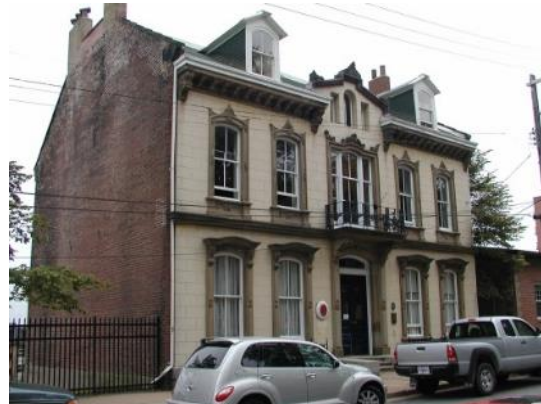
Benjamin Wier House on Hollis Street with prominent cornice and stringcourse
