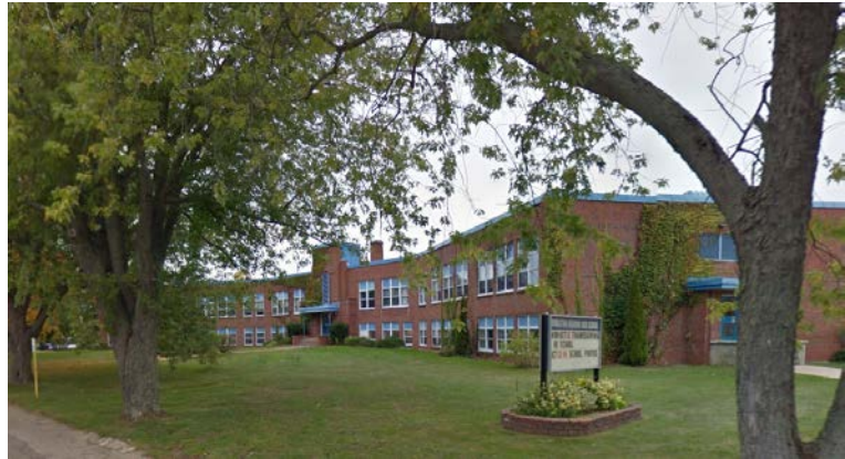
Figure 3: Middleton Regional High School, 2015 (Google Maps)
