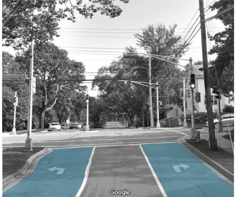
Note that double-left or double-right turning lanes should be counted as **one** turning movement with a turning lane. This is because double turning lanes serve to improve queuing and capacity at an intersection, not safety.
